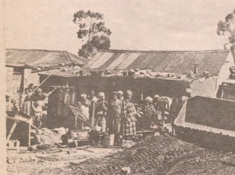
Pimville residents watch their homes being demolished
