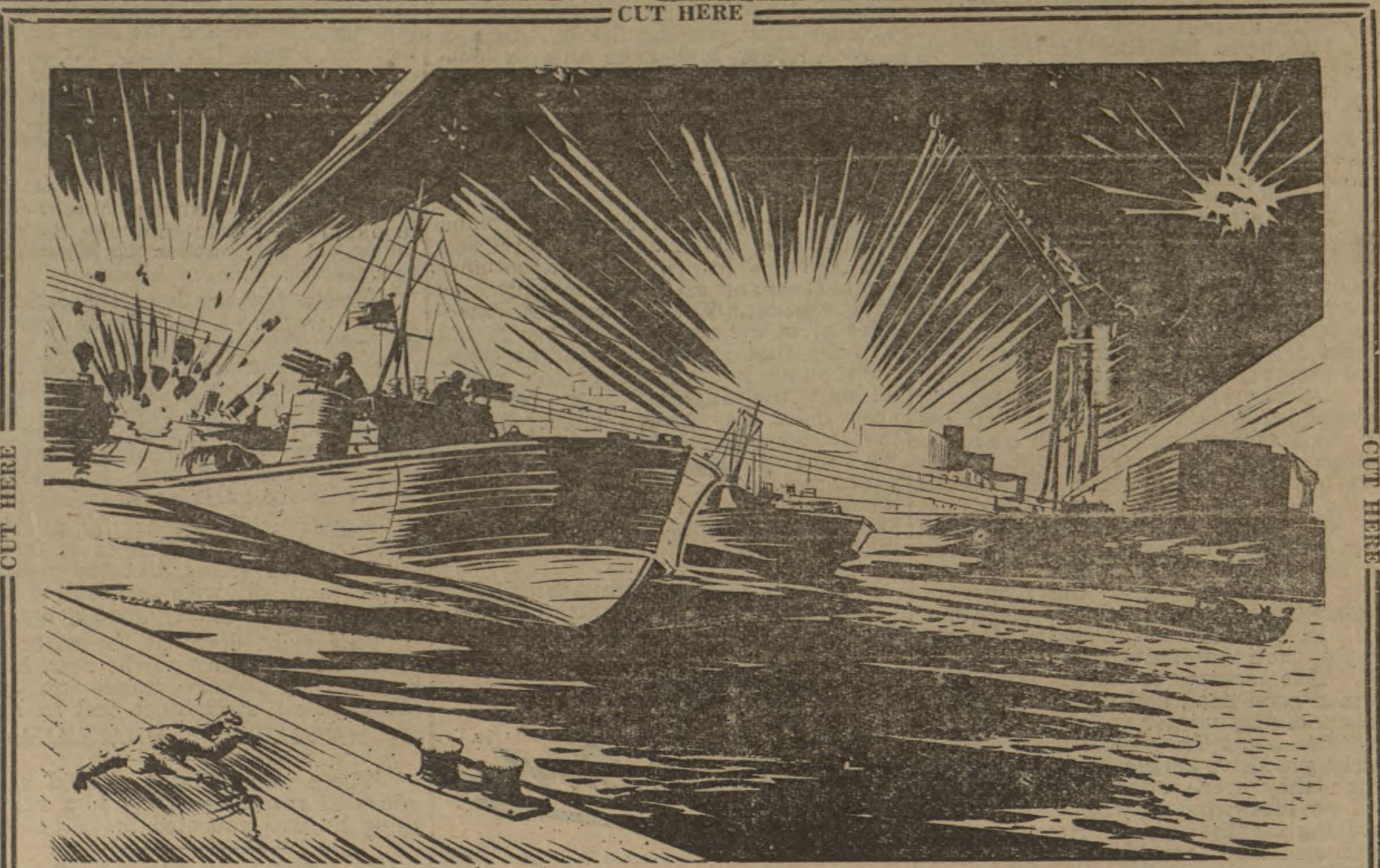
One dark night, British ships sailed right up into the Harbour of St. Nazaire, in German occupied France, blew up the dock gates, destroyed the harbour facilities and burned down many ware-houses. This dangerous piece of work succeeded, and here is one port where the German submarines will no longer be able to shelter.
