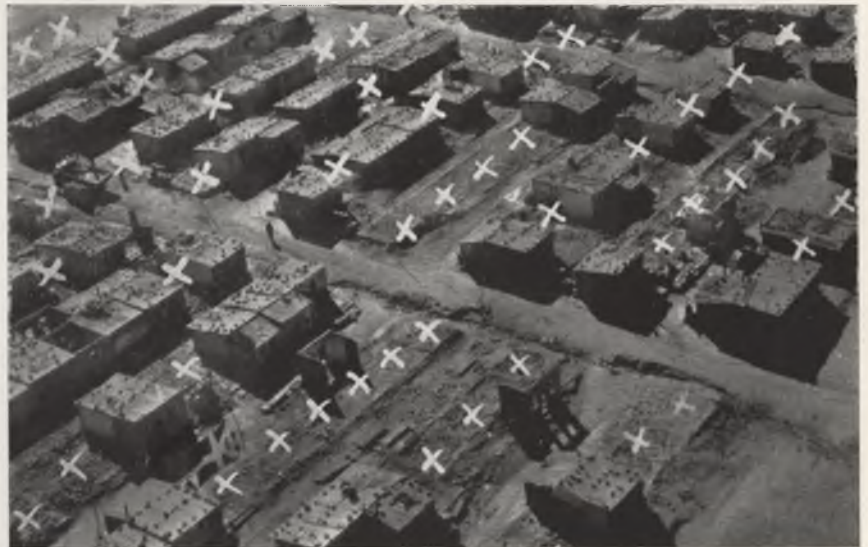
SLUM IN COURSE OF OBLITERATION. As this picture shows, each shack is demolished as soon as its occupants are moved to their new home. Some 70 families have been moved from the small area depicted alone. The sites of demolished shacks are marked by white crosses.
