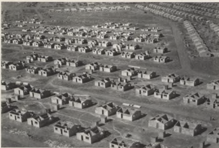
VILLAGE IN THE MAKING. In this Nguni village called Dhlamini houses have been built end-on to the road. Apart from breaking the monotony this practice gives half the houses in any given area added privacy in that their windows face the windowless ends of neighbouring houses.
