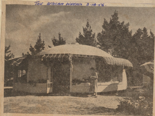
This picture shows the outside appearance of one of the houses being proposed to be built in S. Rhodesia. As you can see it has a round roof and round wall. A special oblong frame is used for the windows. Read the Detailed memorandum and the ground plan on Page 12 of this issue.
