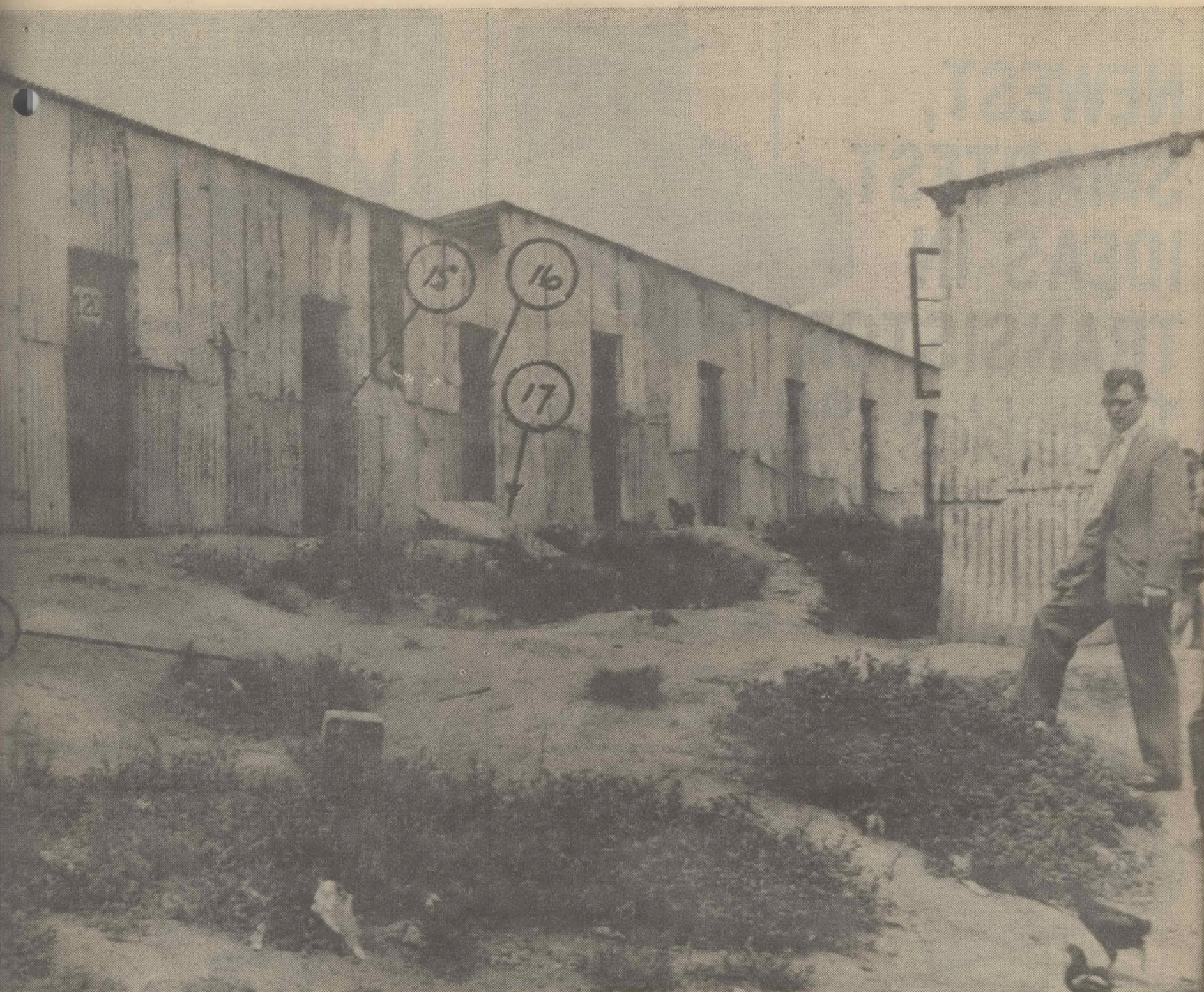
This was the grimy slum-spot where at least three policemen met their death. In doorway 15 the body of Constable Nzuzza was found. Next door, in 16, Constable Rheeders had collapsed unconscious. He survived the attack. Outside at 17, Constable Dhludhla was found and a few feet further away was Sergeant Bhulalo, 18, both were battered to death.
