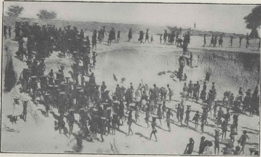
Dam No. 18.—Work in progress.
