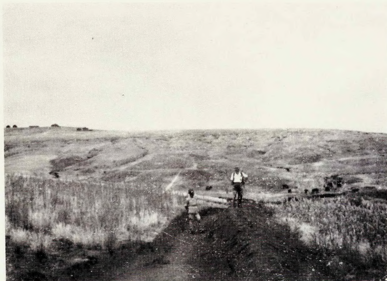
Construction of a diversion furrow
