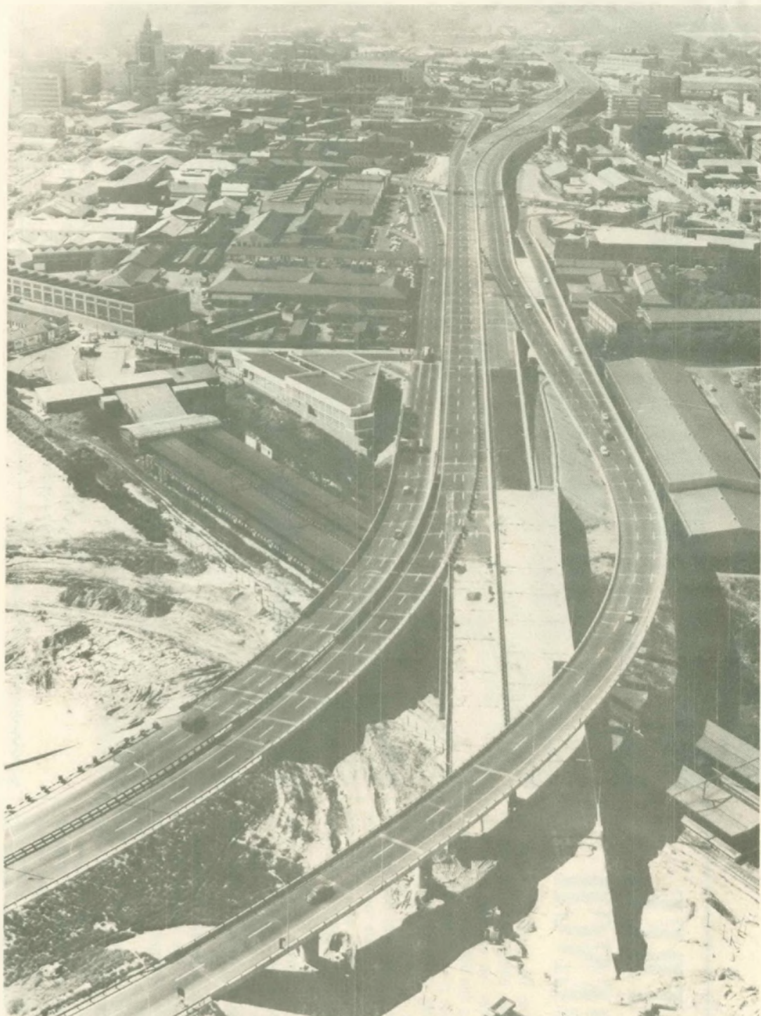
The Westgate Interchange looking east towards the Heidelberg Road Interchange (top right). Between the two interchanges can be seen the central section of the M2 Motorway which was opened during mid-August.
