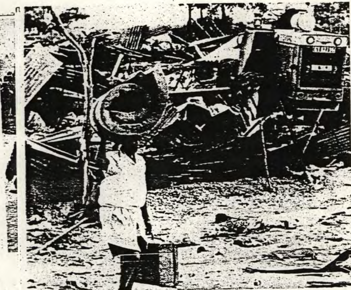
The demolition of Unibel, Cape Town
