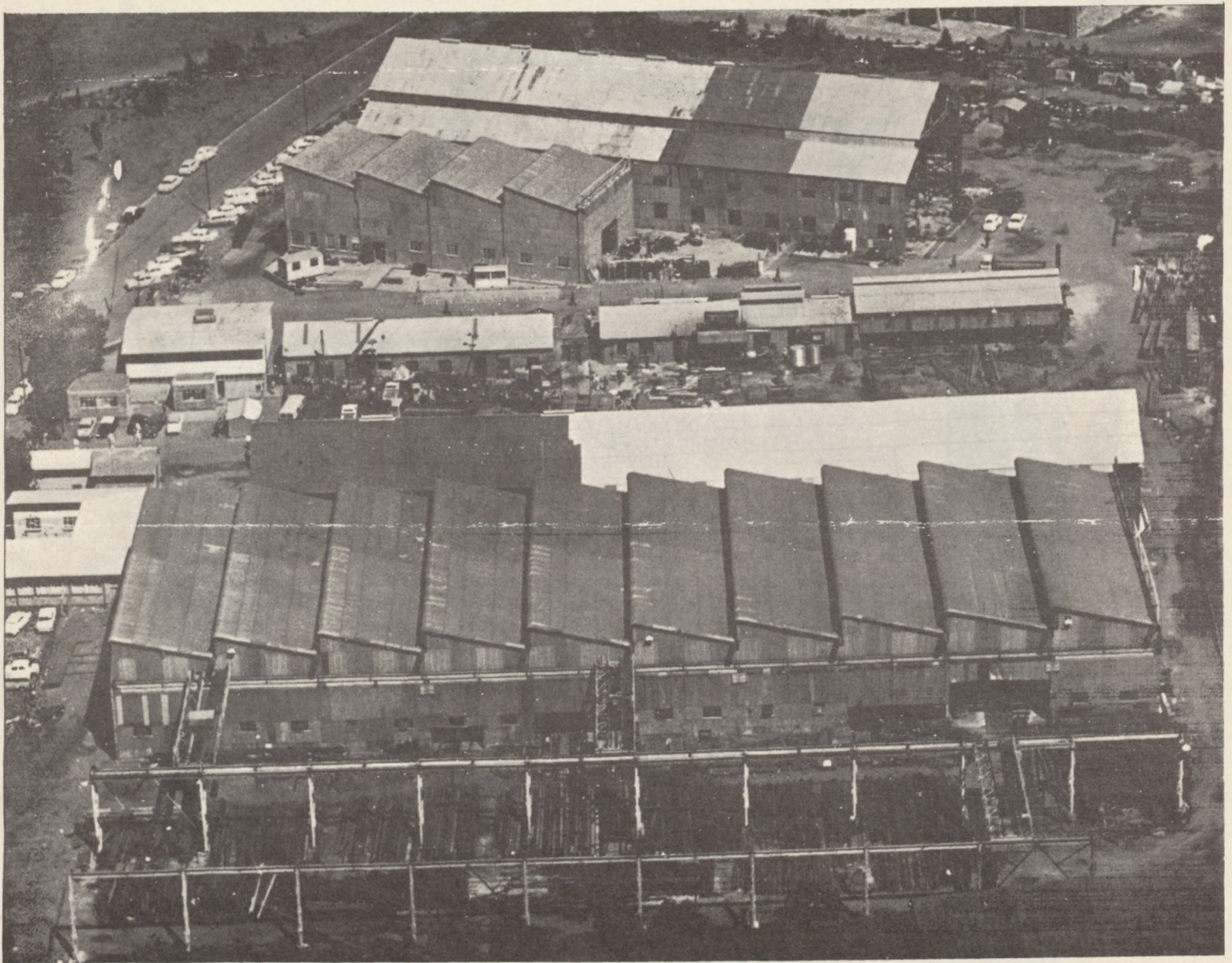
Aerial view of General Erection Co. (Pty) Ltd. at Wadeville, Germiston.
