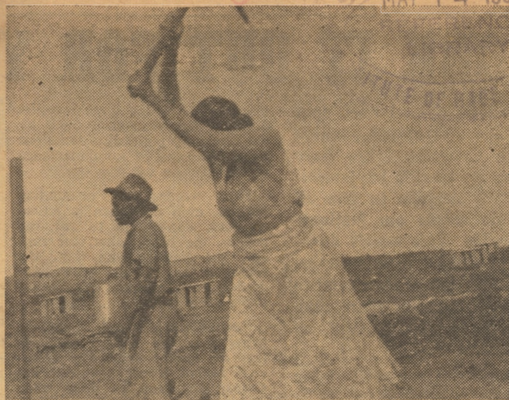
A woman wielding a pick-axe to dig holes for her shanty. Note the latrines in the background.
