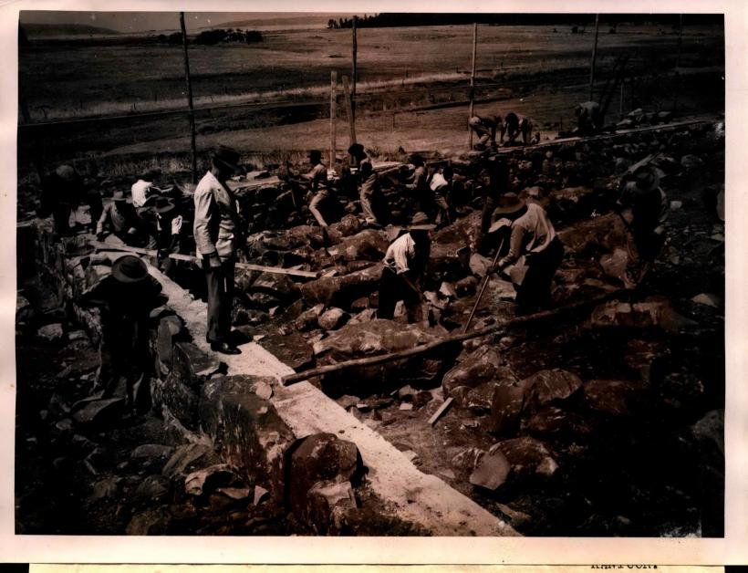
VLAKFONTEIN INDUSTRIAL SCHOOL: BUILDING STUDENTS AT VLAKFONTEIN WORKING ON THE FOUNDATIONS OF THE PRINCIPAL'S RESIDENCE. SOME ARE WORKING ON THE MASONRY FOUNDATION WALL, WHILE OTHERS ARE CLEARING BOULDERS FROM THE SITE WHERE THE FLOOR WILL EVENTUALLY BE LAID.
