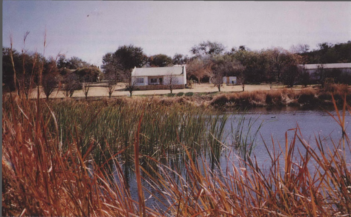
The Retreat and Conference Centre which Robert and Diana Gilbert have built at Ridor Reitfontein.
