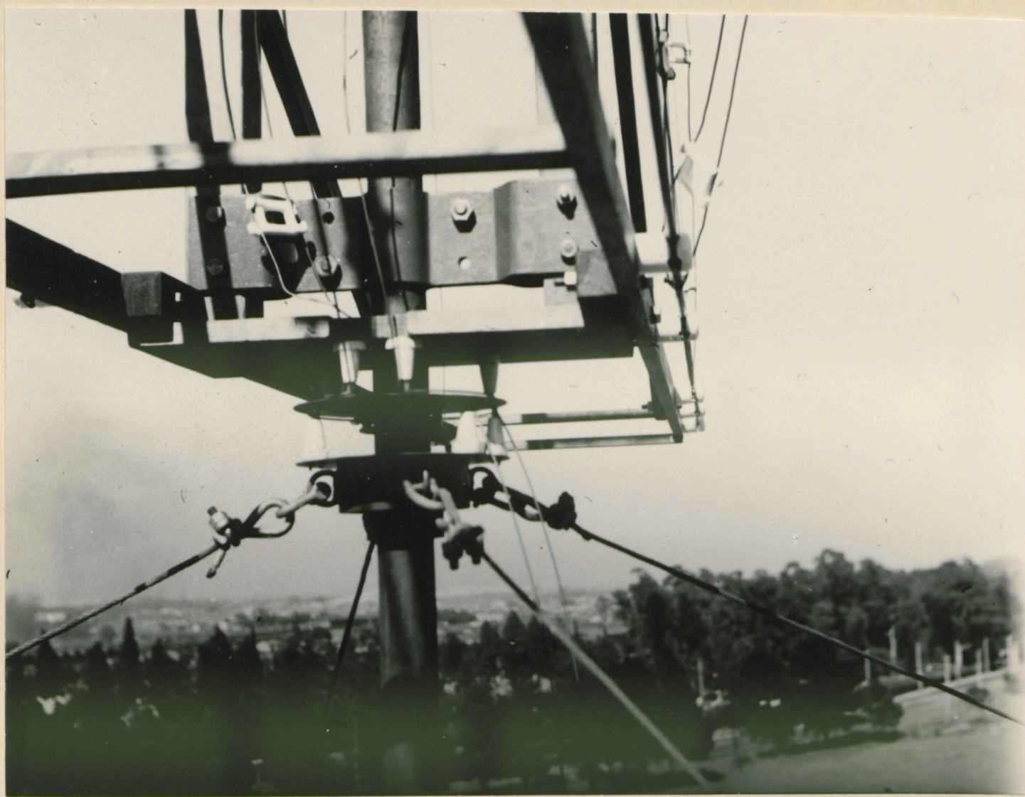
ROTATING COUPLING ASSEMBLY ON THE AERIAL POLE.
