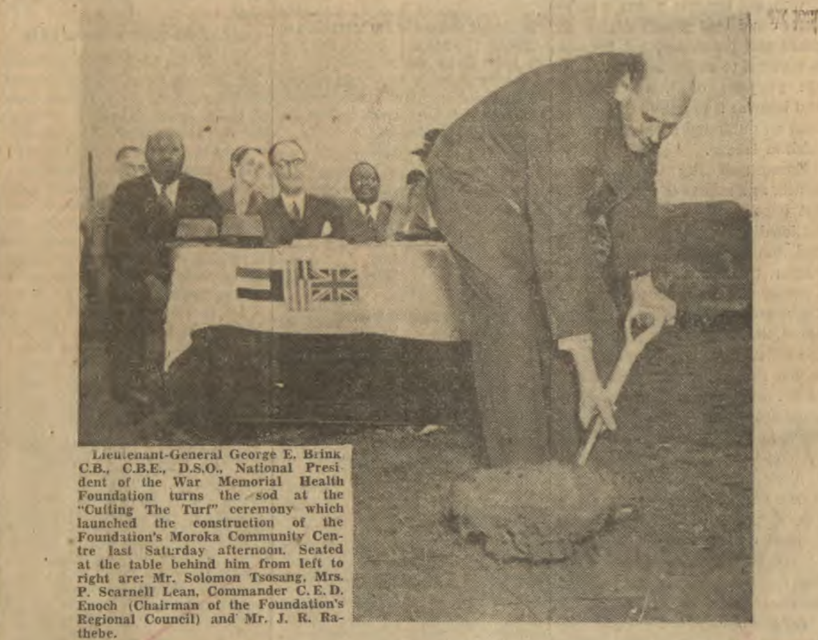
Lieutenant-General George E. Brink, C.B., C.B.E., D.S.O., National President of the War Memorial Health Foundation turns the sod at the "Cutting the Turf" ceremony which launched the construction of the Foundation's Moroka Community Centre last Saturday afternoon. Seated at the table behind him from left to right are: Mr. Solomon Tsoang, Mrs. P. Scarnell Lean, Commander C.E.D. Enoch (Chairman of the Foundation's Regional Council) and Mr. J. R. Raathebe.
