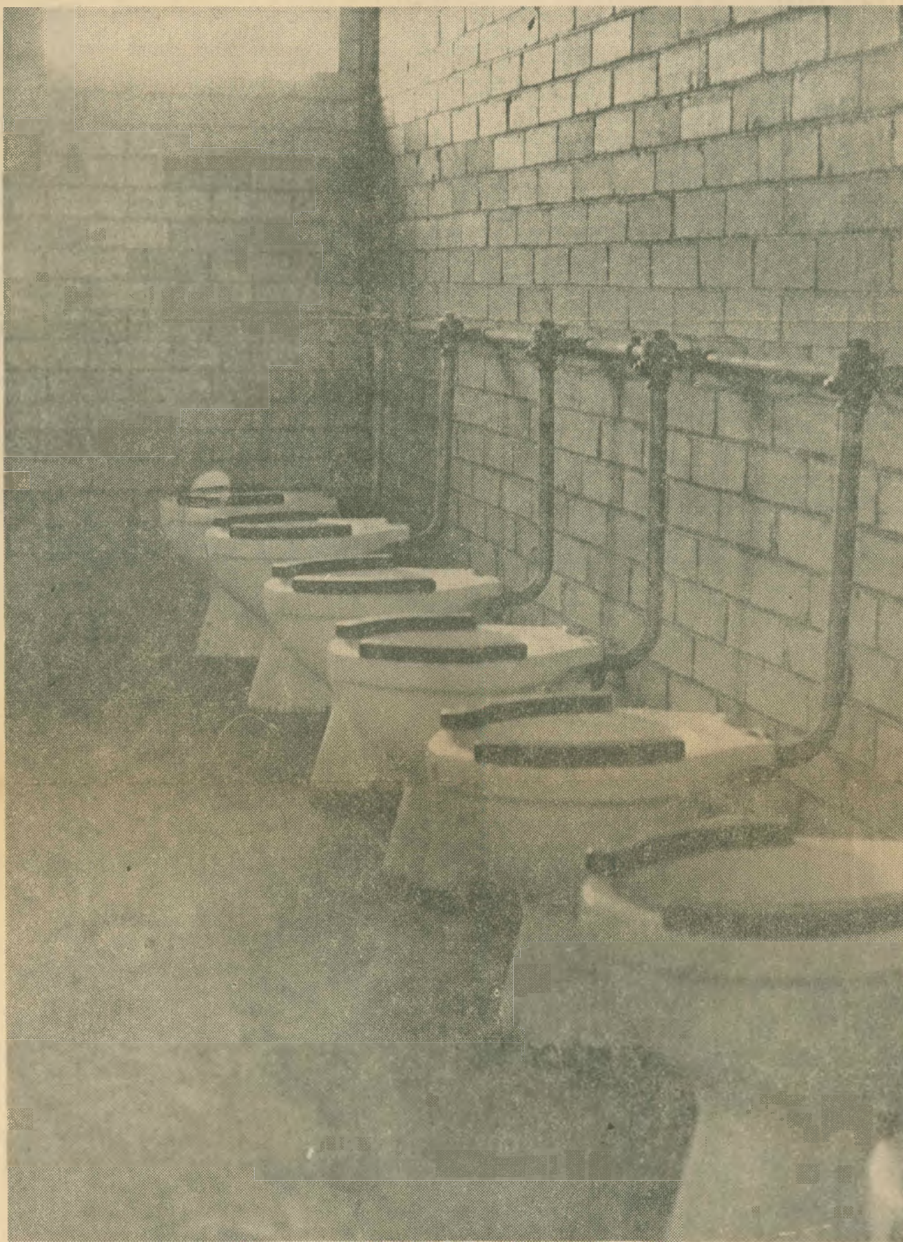
Toilet facilities at the Diepkloof Men's Hostel.
