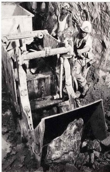
A shovel loader clearing broken rock in a development end at the Western Deep Levels mine
