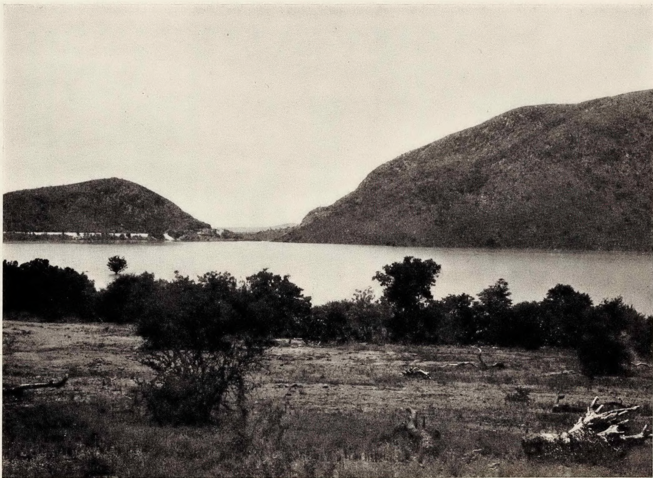
Photo: S.A. Railways and Harbours. OLIFANTSNEK DAM, Rustenburg, Transvaal.
