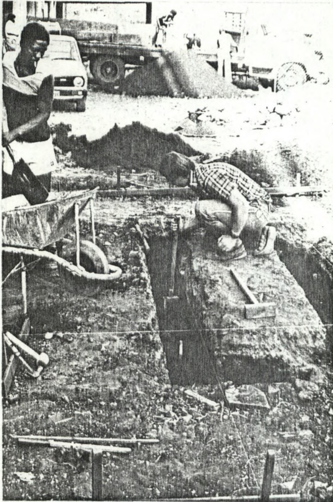
TRADITIONAL FOUNDATION EXCAVATION
