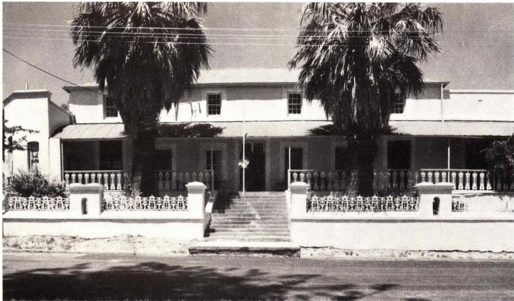
1 Kerkstraat nr 42 na die aardbewing in 1969. No 42 Church Street after the earthquake in 1969.
