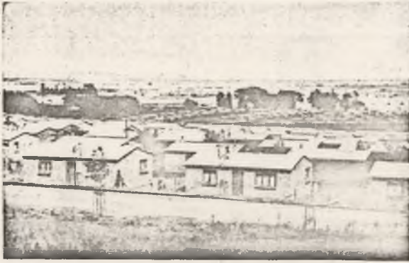
Completed houses for Bantu in Dube Township.
