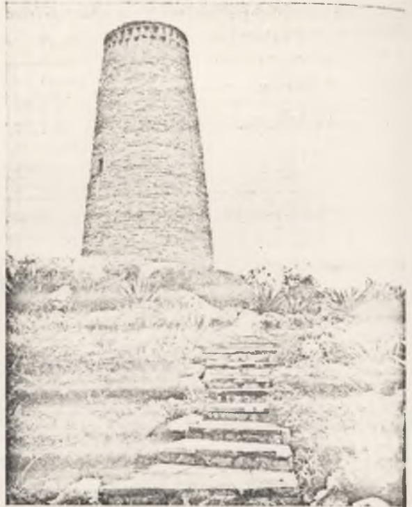
Constructed from materials used for the 'building' of shacks and lean-to's in Shantytown, the Oppenheimer Memorial Tower, Soweto, erected to the memory of the late Sir Ernest Oppenheimer.
