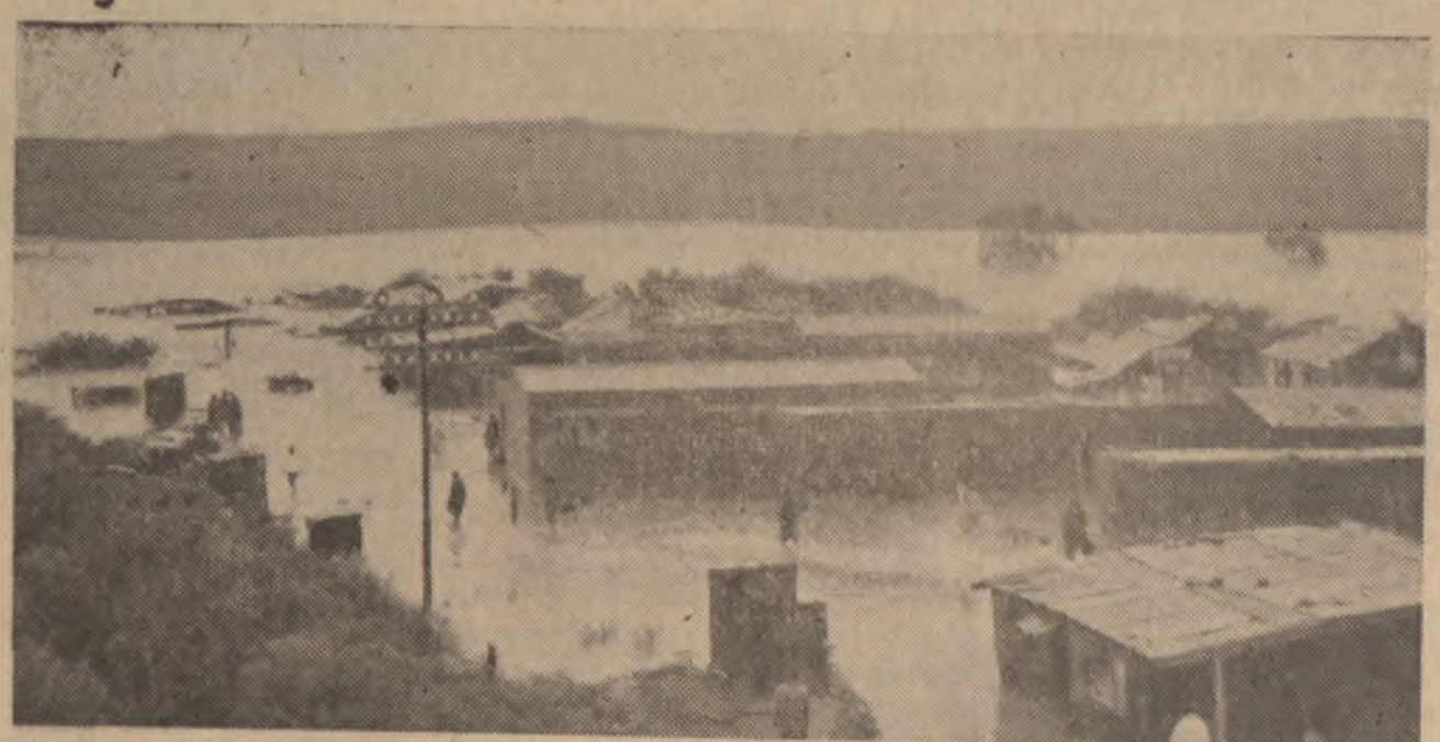
The township of Kliptown was flooded last week as the result of the heavy rains that fell throughout the Transvaal. Many houses collapsed, and their owners are accommodated in tents supplied by the military authorities.
