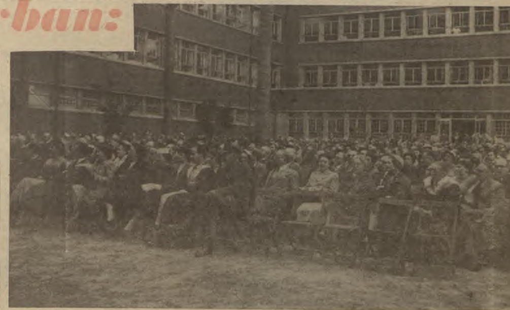
ABOVE: A section of the audience of 2,000 guests present at the opening of the Medical School in Durban. Part of the superb new building can be seen in the background, with the palm trees of Durban in the courtyard. There are many windows so that the students can work easily, with good light.
