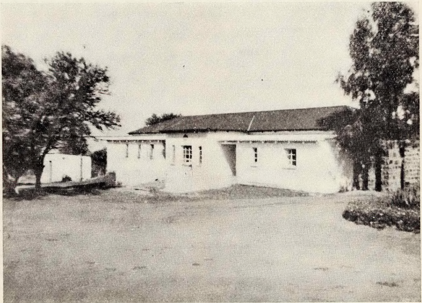
St. Anne's Maternity Department nearing completion.
