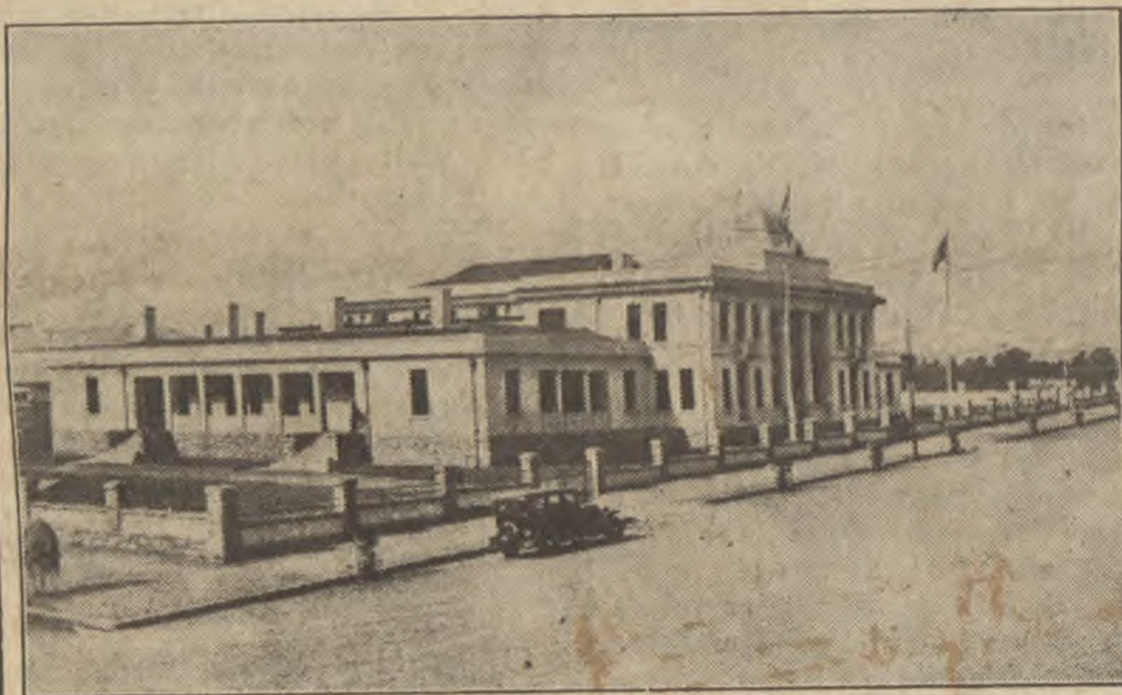
The Bhunga Buildings at Umtata, Transkei.
